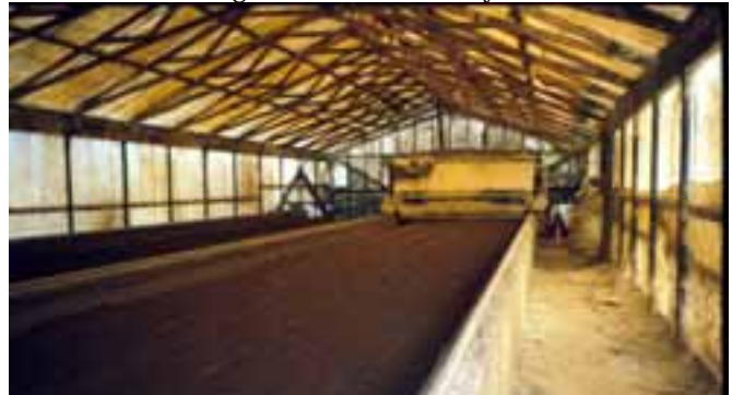
Bed Composting System
