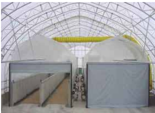
Bay Composting System
