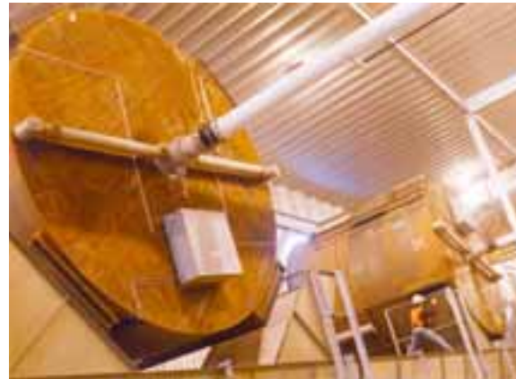
In-Vessel Aerobic Composting
