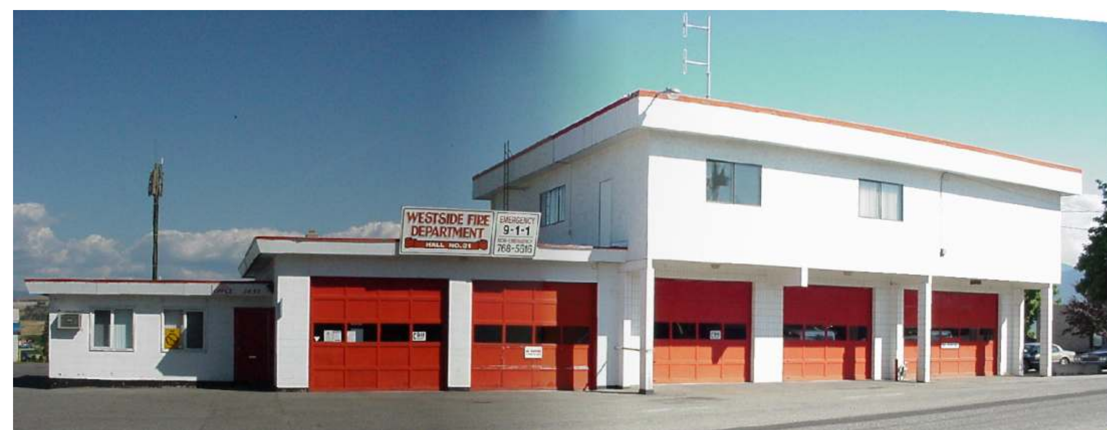
Westbank Main Hall 3651 Old Okanagan Highway
