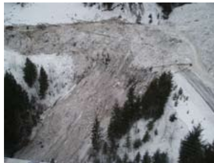
Avalanches taking powerlines down.
