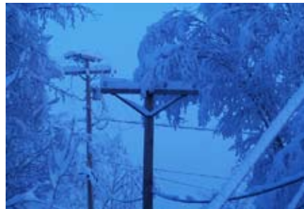
Trees with heavy snow drooping onto powerlines.
